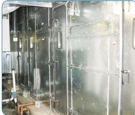
**Assembled 38,000 cfm Ventrol AHU that was brought into a tight quartered equipment room through a 60-inch x 60-inch square opening.**
